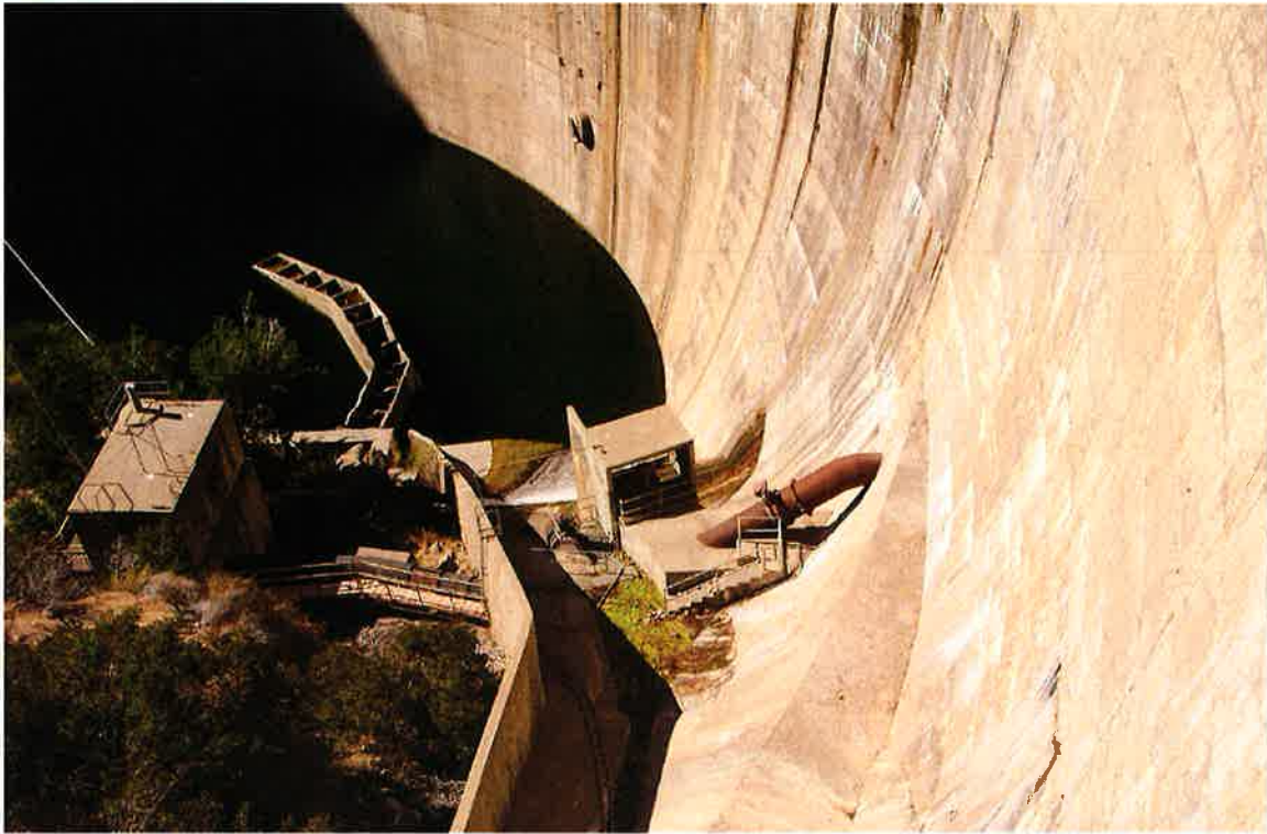
12. View of the outlet works at downstream toe of dam.
