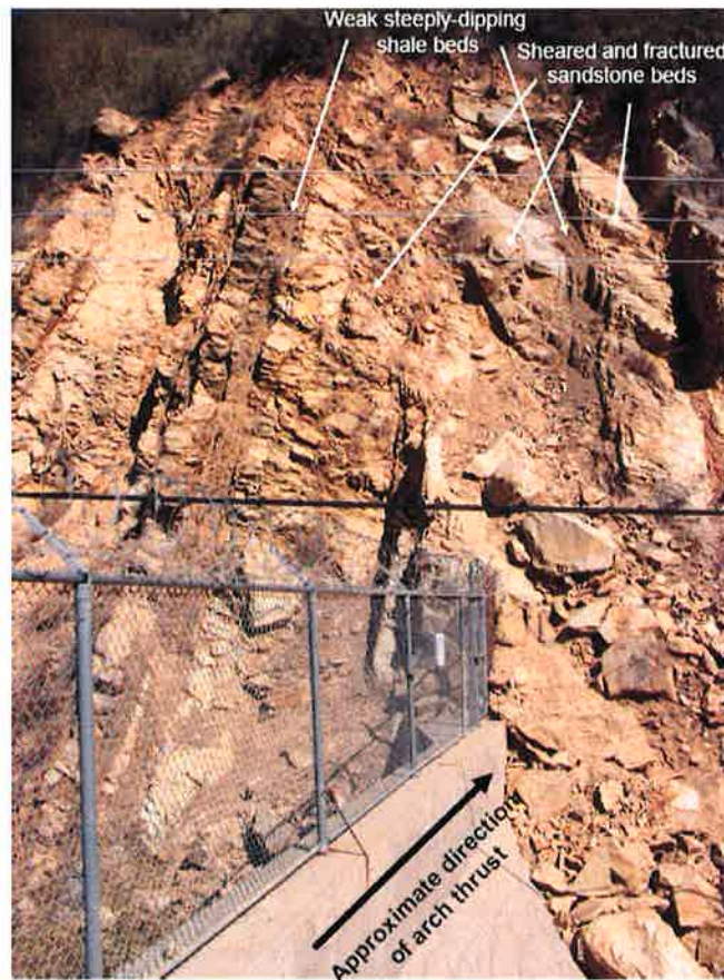
Weak Rock in Left Abutment
