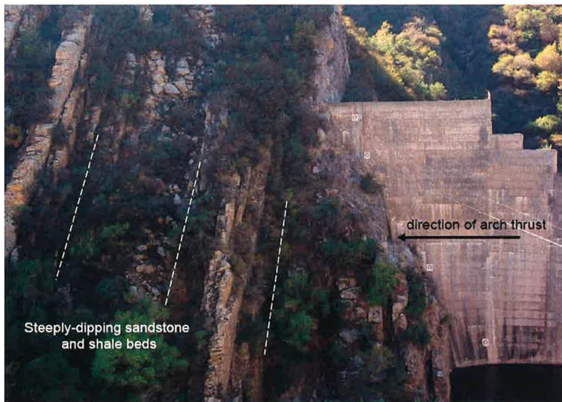
Steeply-Dipping Rock in Right Abutment
