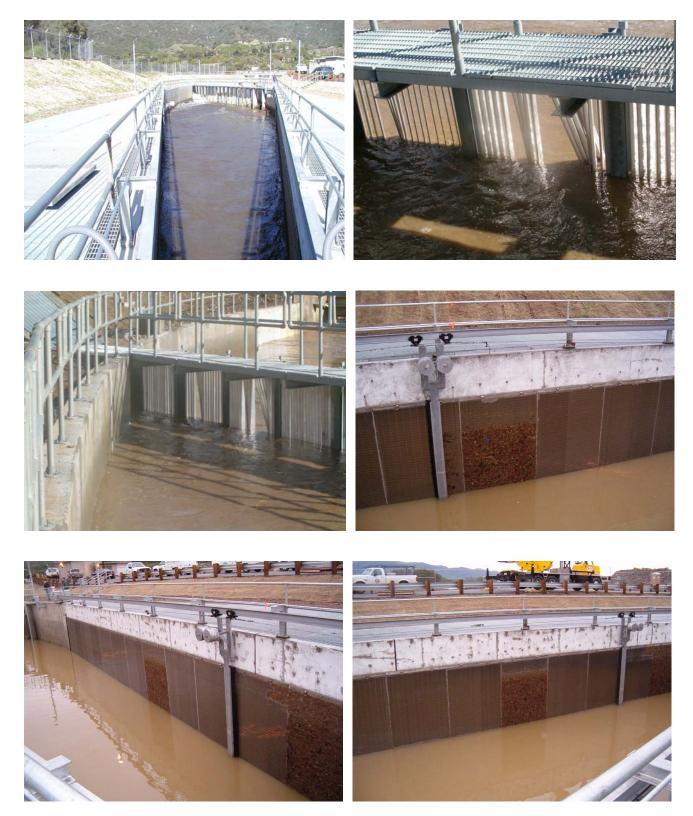
1/03/05 – Damage to fish guidance device resulting from flow entering facility and the collection of plant debris on the facing of each fish screen. Brush system failed to operate during this storm event.
