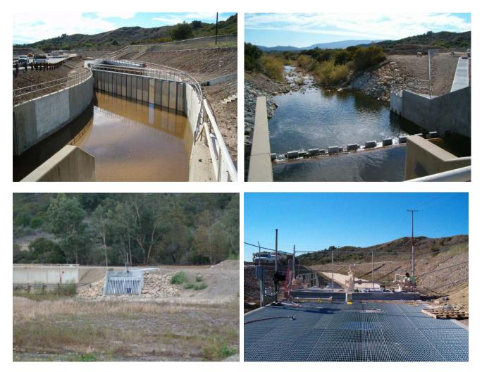
11/3/04 – Small amount of runoff allowed to pass through the spillway gates while work is proceeding in the fish passage and on the overshot gate (top and middle).
