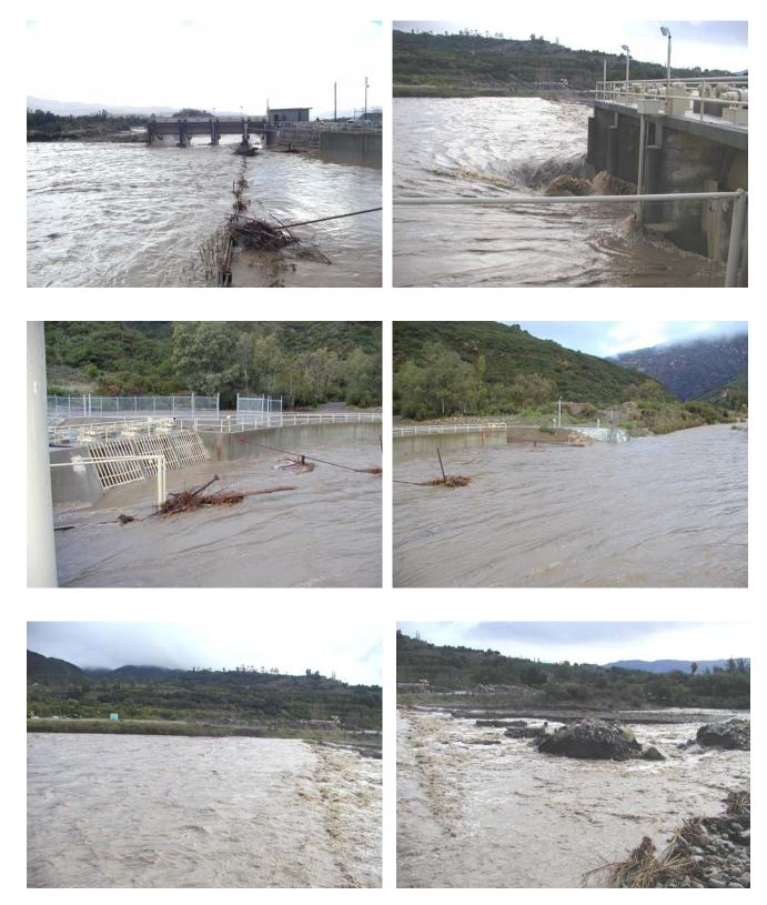
12/31/04 – Robles Basin conditions during the first major storm of the season. Trash wall and spillway gates (top left and right), Canal Entrance (middle left) and fish exit structure (middle right), and Robles basin and cutoff wall breaching (bottom left and right) during peak of storm.
