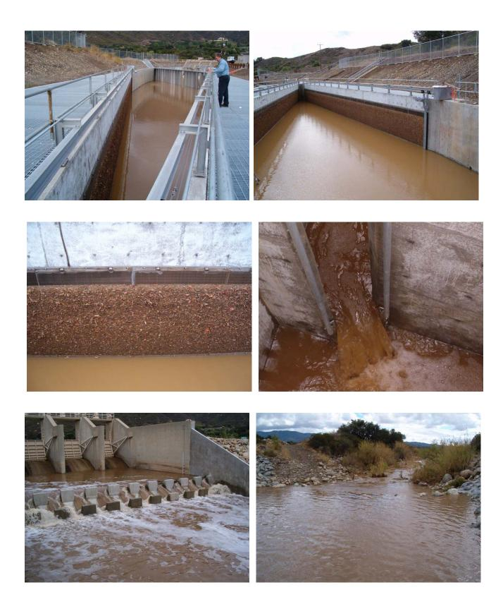
10/20/04 – Early storm runoff that caused a collection of vegetation debris on the face of the fish screens (middle left), near complete plugging of screens. Flow filled the upstream basin and caused overflow at the cutoff wall. When discovered, release made through spillway gates (bottom left) to downstream channel (bottom right).
