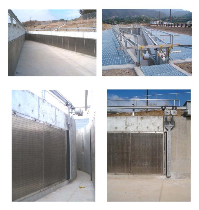
10/1/04 – Project construction continuing with the installation of fish screens and brush system. Note that the electrical and programming systems for the brush system were not installed until the last week of December 2004.
