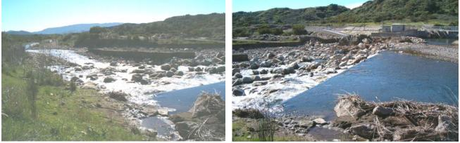
Aftermath of 1/10/05 storm event – damage to fish guidance device, sediment loading in the upstream basin that cut off flow to Fish Passage Facility. (Photos not taken during the peak event due to emergency in other areas.)
