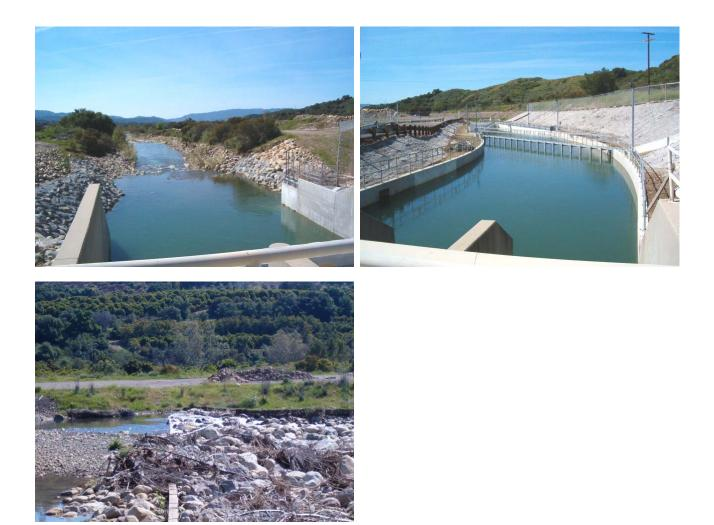
3/25/05 – Facility in operation without the use of the fish guidance device, water flowing over the cutoff wall.
