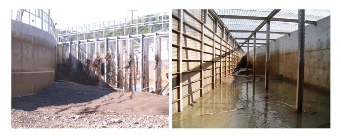
3/03/03 – District performed maintenance on the fish passage facility. Sediment deposition in the forebay.
