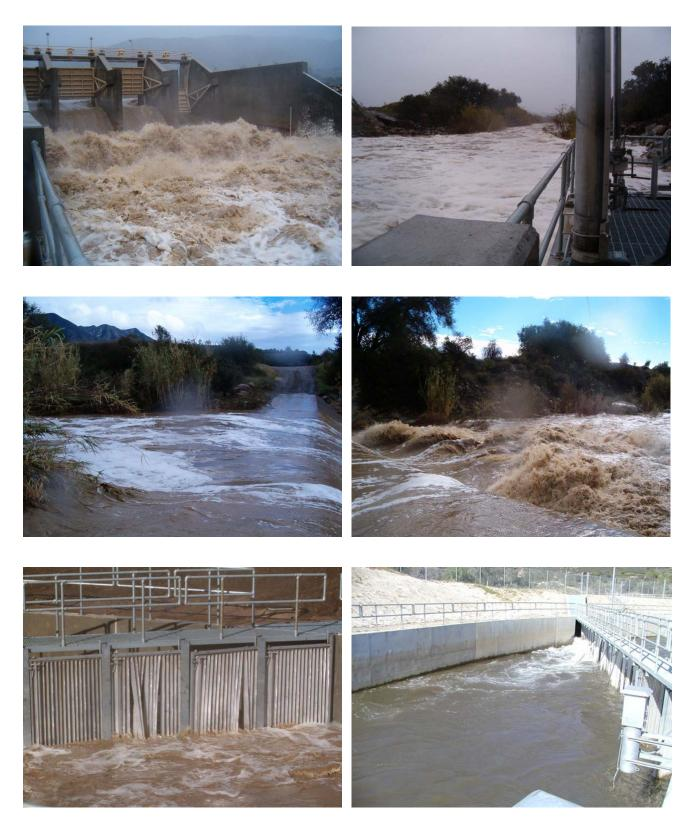
1/3/05 – Storm flows through Robles spillway gates and downstream channel (top), over the measurement weir (middle) and damage to fish guidance device (bottom).
