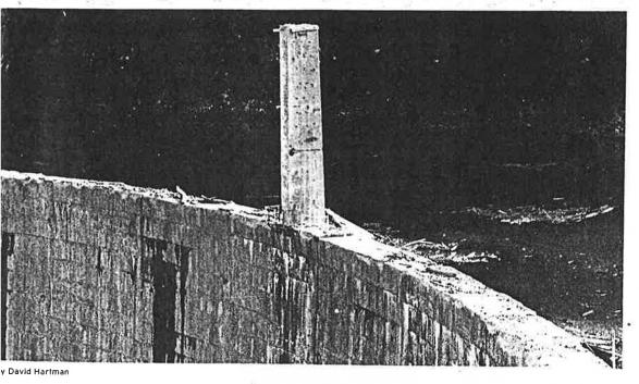
A no longer-functional cement structure on top of Matilija Dam, left, is destroyed by a dynamite blast, below. The blasting is part of repair work being done by the Ventura County Flood Control District that will allow workers to release water through the dam without having to walk out to the cement tower that once supported bridges and mechanical equipment.
