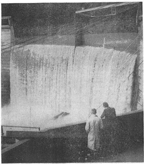
OVER THE TOP — The <u>Matilija Dam</u> northwest of Ojai, nearly empty last night, began spilling water this morning at 3 a.m. when a cloudburst hit the area. The water spilled over the notches cut in the dam late last summer to insure that the dam would be safe.
