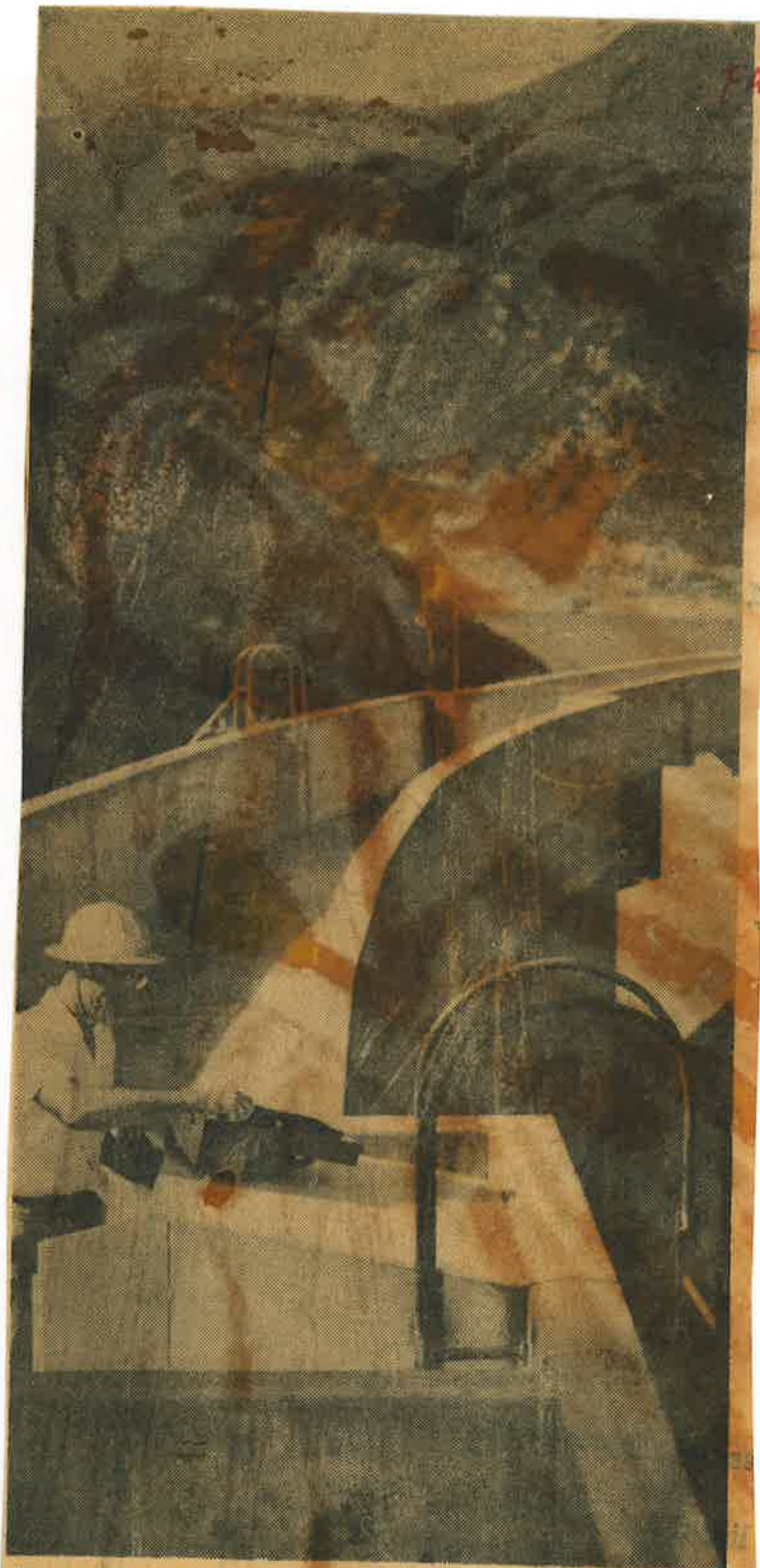
George Gonsman, engineering technician for the Water Resources Division of the Ventura County Department of Public Works, periodically takes electronic readings of strain gauges set into Matilija Dam and canyon walls.
