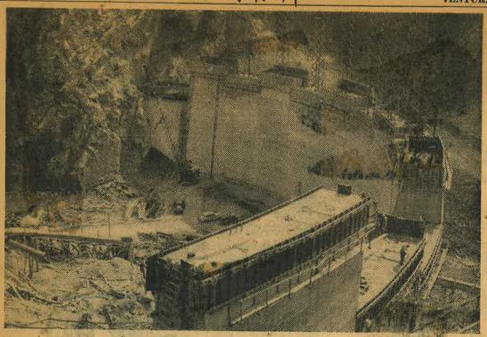
GROWING STEADILY—Matilija dam yesterday had reached an elevation of 1,085 feet in the highest block as workmen continued to rush it nearer completion. At the base of the dam, can be seen a crane with a 100-foot boom which is hoisting buckets of concrete into the forms atop the dam. On top of the forms can be seen the trestles which will reinforce the concrete.
