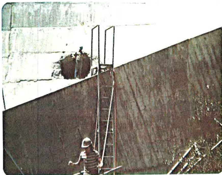
Photo No. 5.7 New 42-inch outlet under construction.
