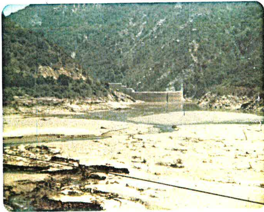
Photo No. 5.1 Dam and reservoir depositions.
