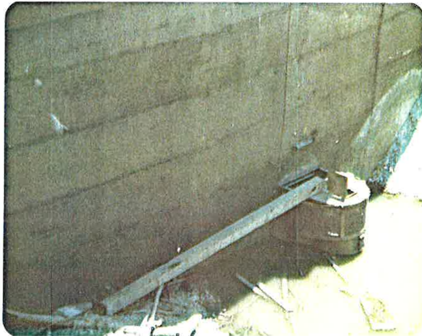
Photo No. 5.8 Outlet intake riser. Note damaged area.
