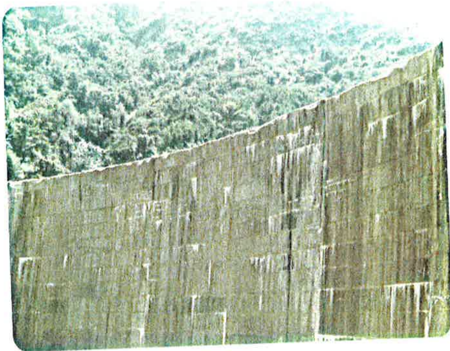
Photo No. 5.4 Center arch. Note crack pattern on lifts and between lifts.
